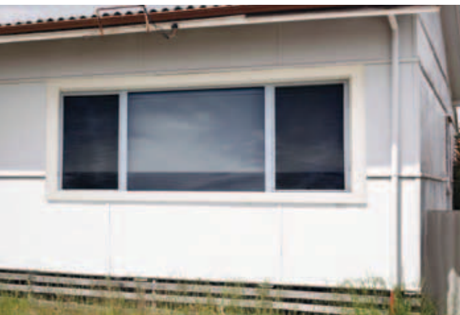
Install maintenance free aluminium sliding windows
